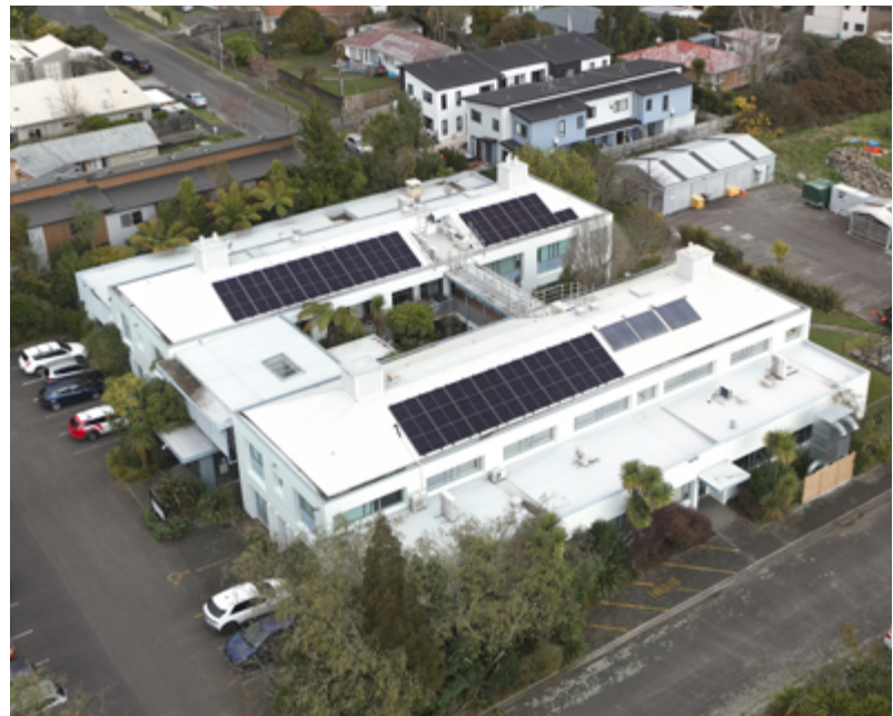
Solar panels on the roof at our Hamilton site.
